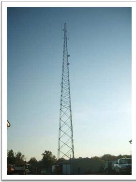
A typical BRICS radio tower includes antennas and microwave dishes. This tower, in Oxford, rises 350 feet.
