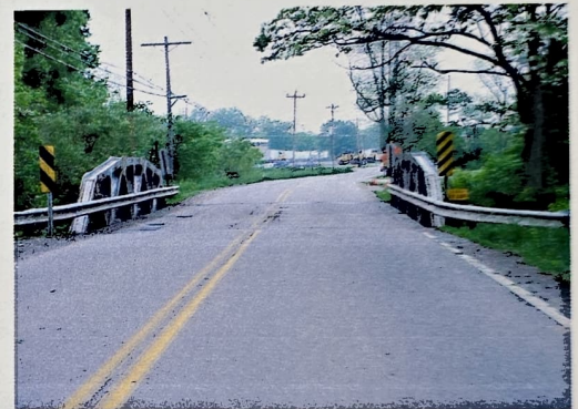
Allen Road Bridge
